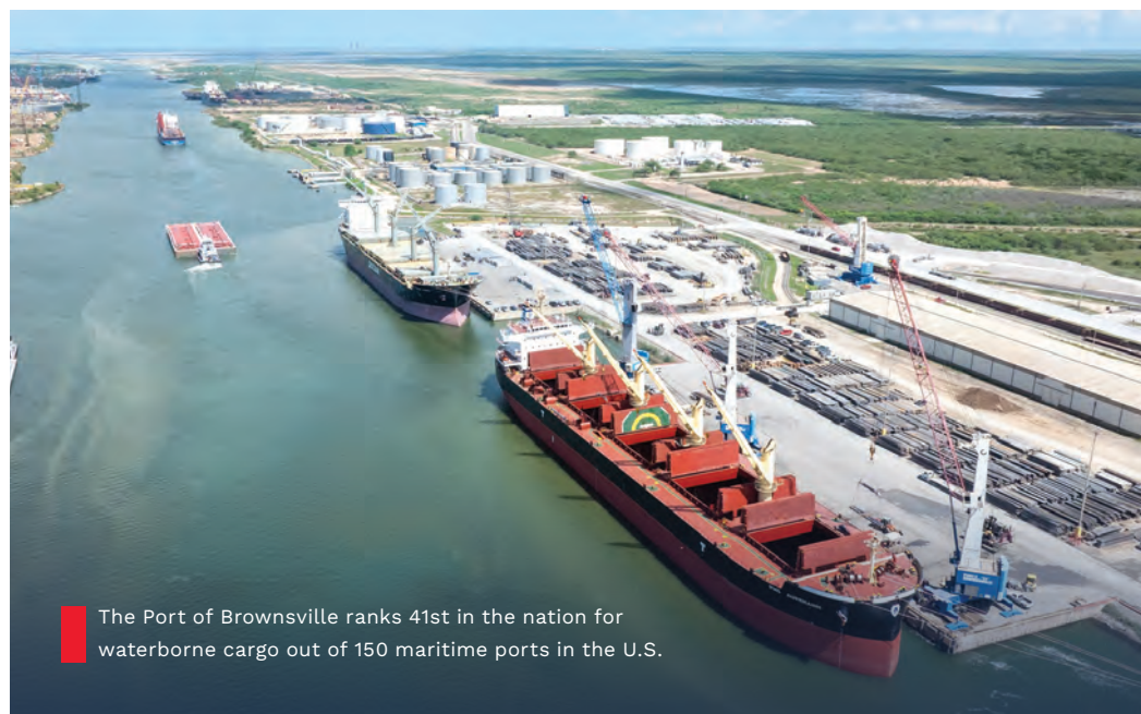
Project cargo for Rio Grande LNG is loaded onto a barge for transport to the LNG facility.
