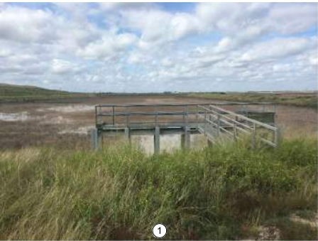
EXISTING OUTFALL STRUCTURE PHOTO
