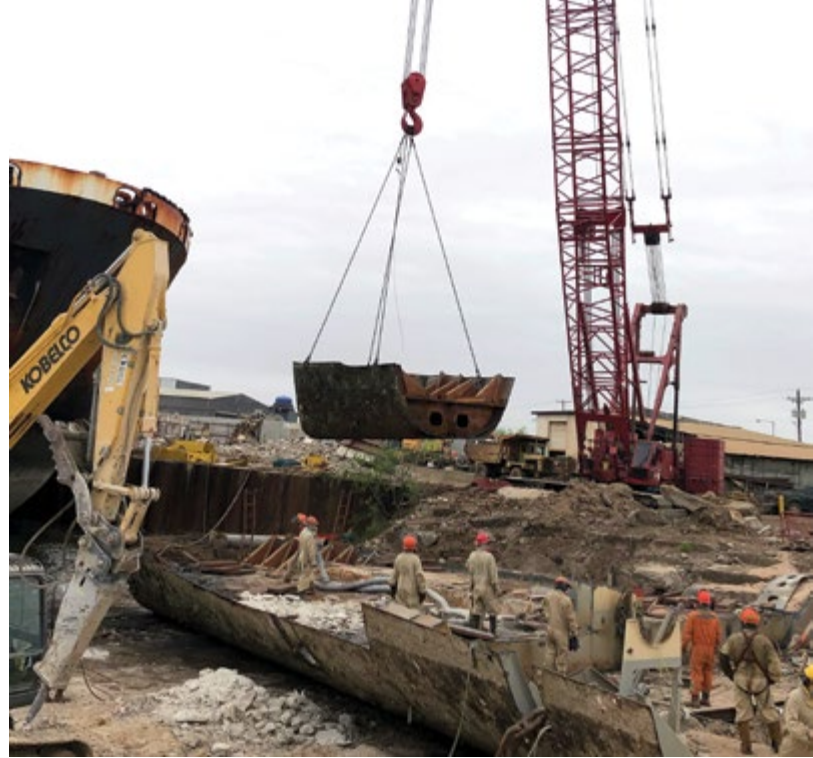
ABOVE – The final piece of the former floating nuclear power barge Sturgis is hauled away March 2019 by International Shipbreaking, Ltd.'s proud workers. Photo courtesy of the U.S. Army Corps of Engineers.
