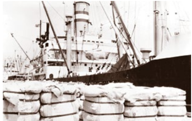
THEN: Early successes at the Port of Brownsville included shipments of cotton and fruits.
